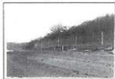
Taken from the shore in front of the blockhouse, looking west. It is possible to see that none of the built up concrete base that people walk along today existed then.
